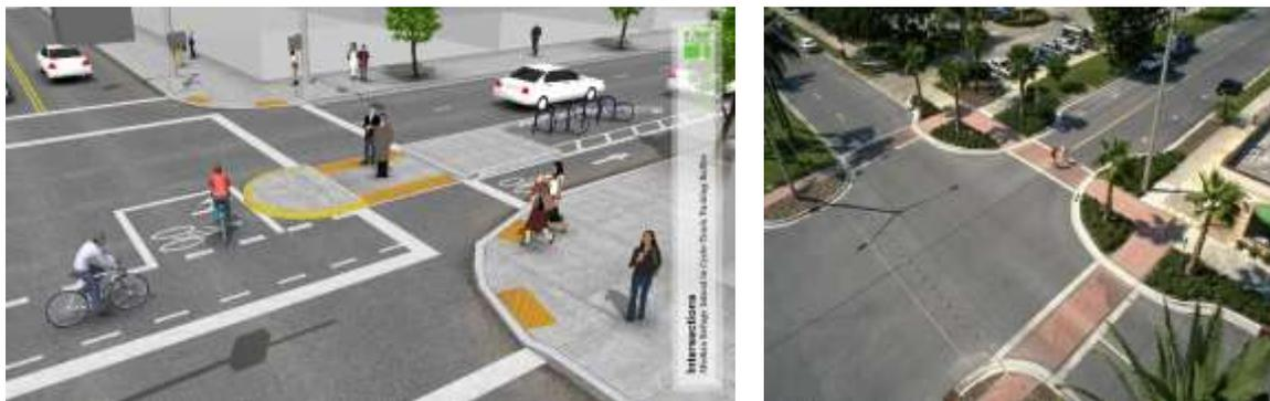
*Figure 2: Median islands and curb extensions are two examples of traffic calming measures.*
